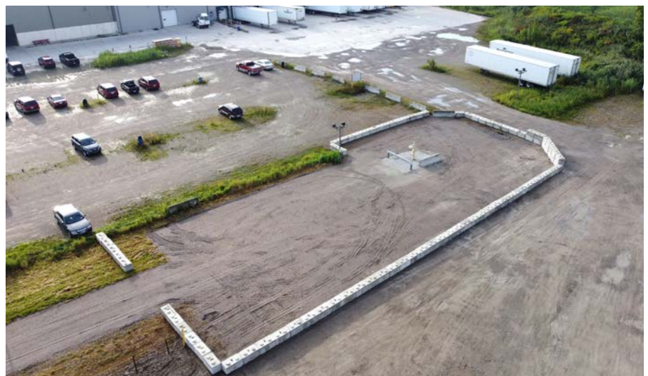
Well Site Protective Barriers - Figure 58
