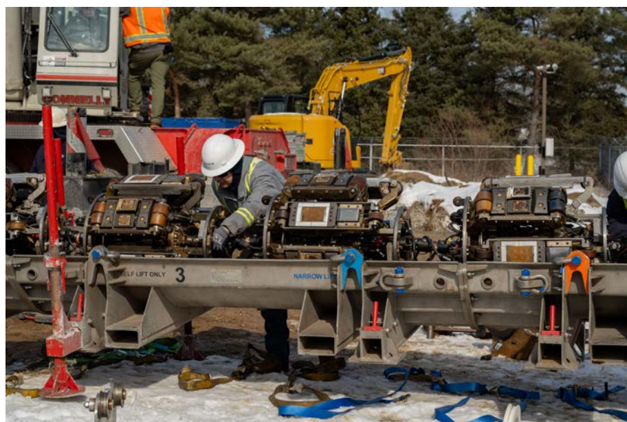
DTE Gas Crew Performing an ILI Inspection – Figure 50
