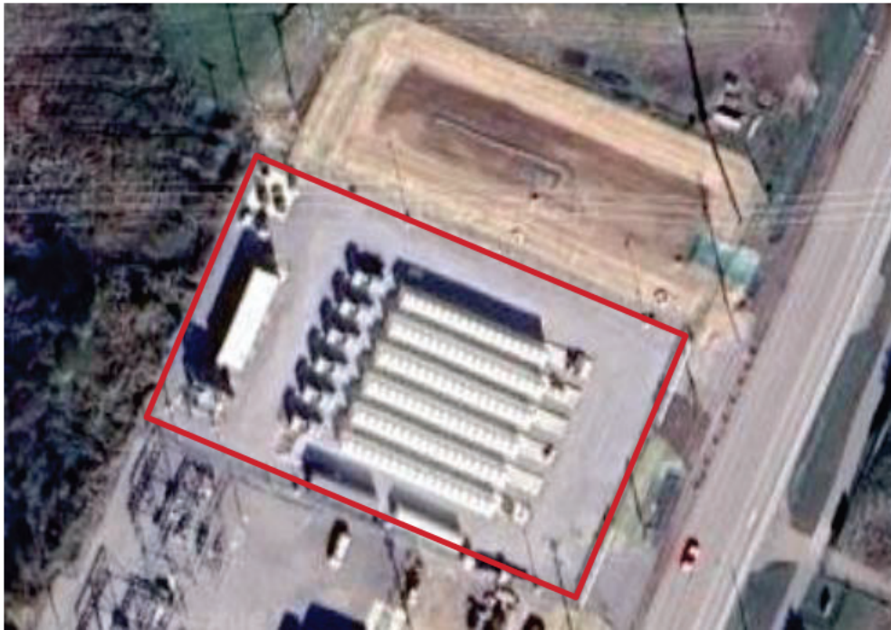
Figure 2-1 — Slocum BESS Aerial View
